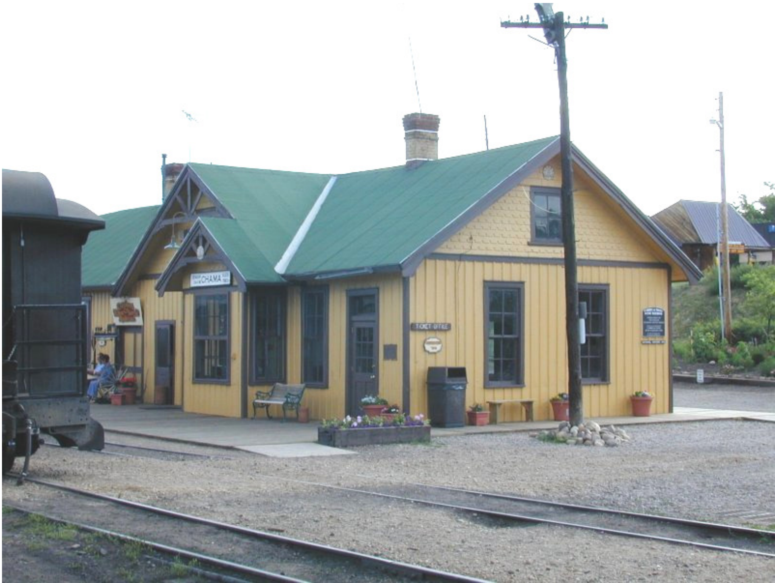
C&T Chama Station
