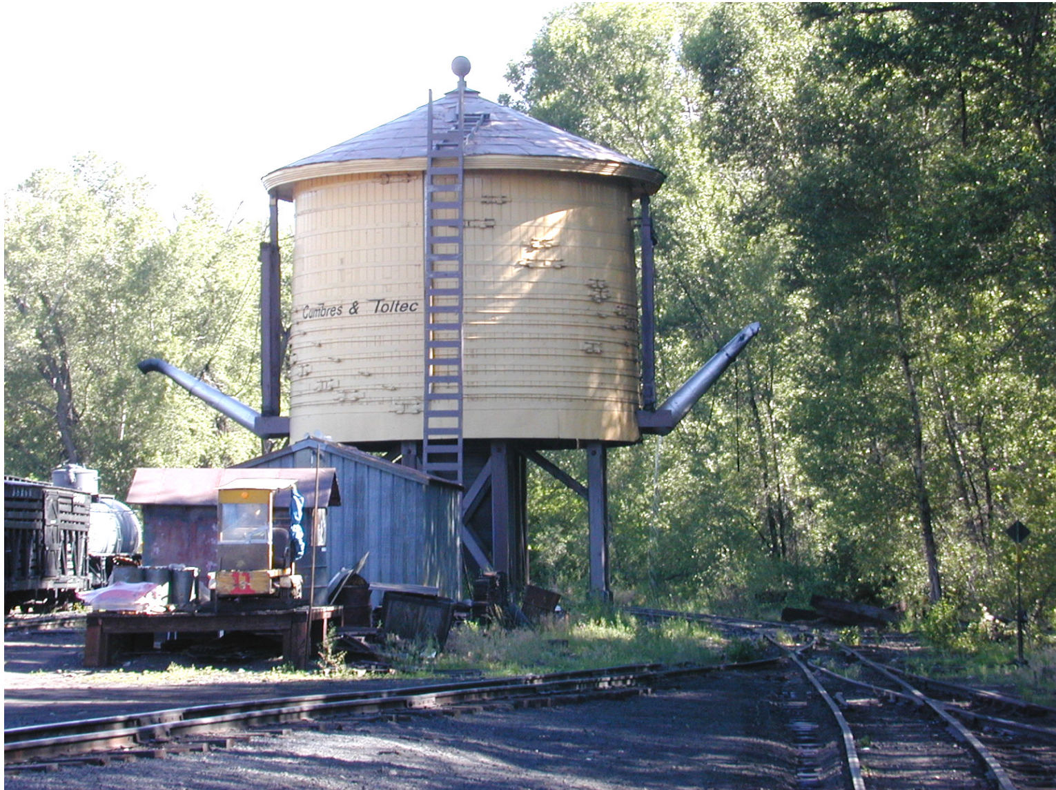
C&T Water Tower
